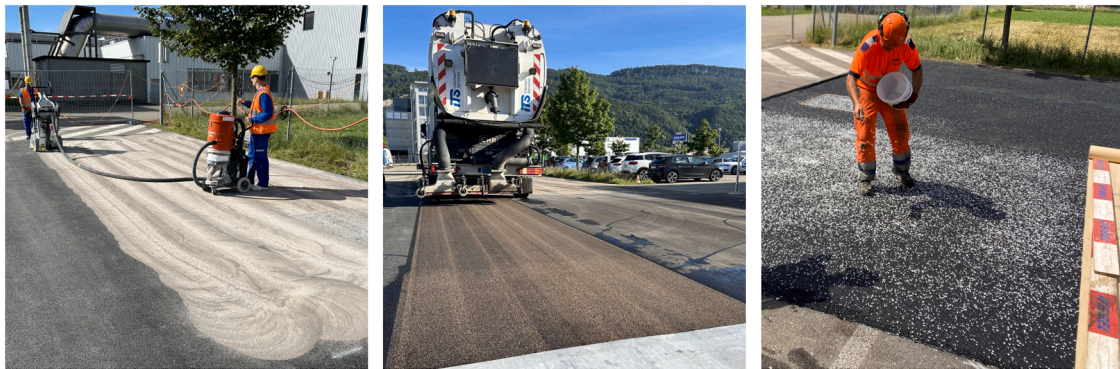
Fig. 2. Surface treatments applied to asphalt pavements: (left) grinding, (center) water blasting, and (right) gritting.
